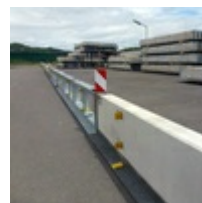
Temporary crash barriers
