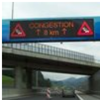
Variable message signs VMS LED
